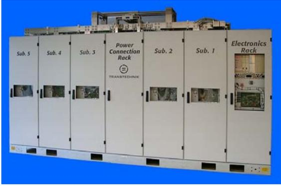
Figure 9. [13kA, 18V] converter
